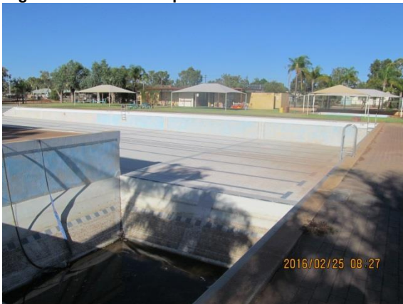
Figure B.3: View of the pool from the north east corner.
