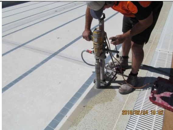
Figure B.43: The core hole at Location 10 on the north west corner of the pool.
