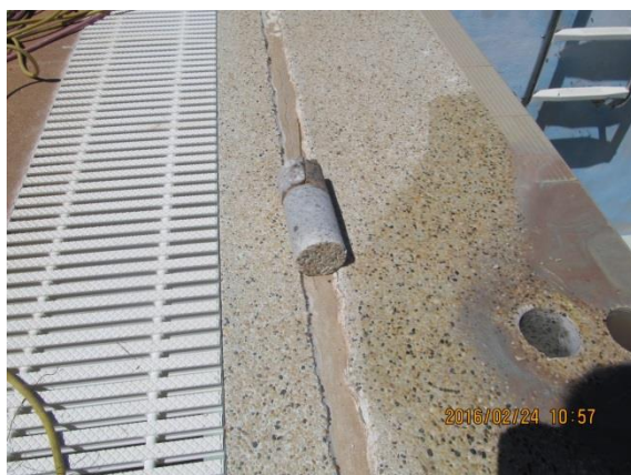
Figure B.47: The core hole at Location 11 on the east side of the dive pool.
