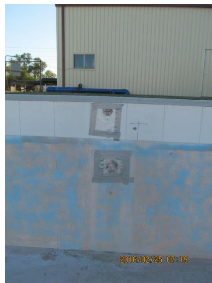
Figure B.34: Repaired core hole 7 taped over with polythene sheet.
