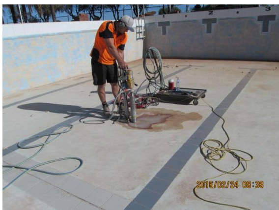
Figure B.35: The core hole at Location 8 close to the north west corner of the pool.
