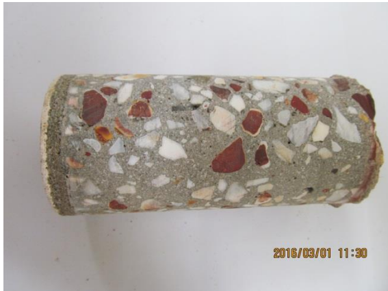
Figure 8: Core 7 Beneath splash zone sample showing the white topping and intermediate material over the concrete with multi-coloured aggregates.
