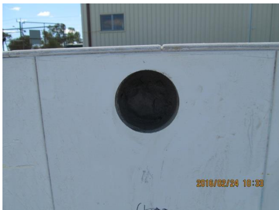
Figure B.23: The core hole at Location 5 on the east side of the pool.
