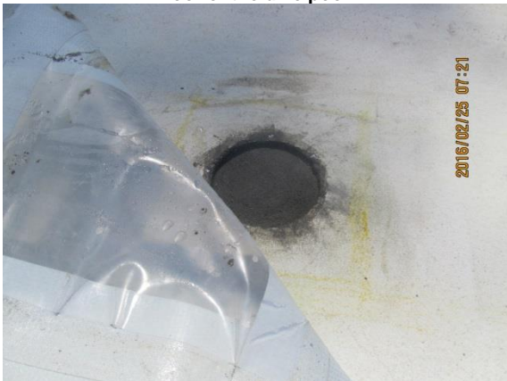
Figure B.53: Repaired core hole 12 after curing overnight.
