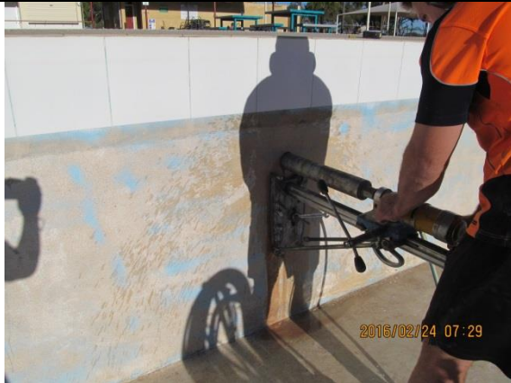
Figure B.55: The core hole at Location 13 on the west side of the pool.
