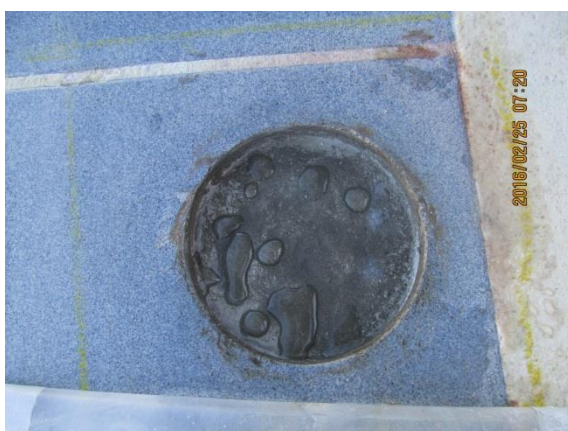
Figure B.29: Repaired core hole 6 after curing overnight.
