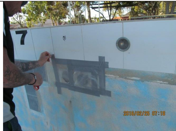
Figure B.14: Repaired core hole 2 taped over with polythene sheet.
