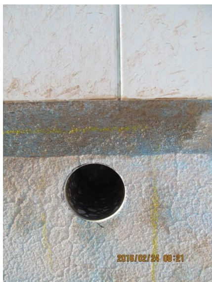
Figure B.11: The core hole at Location 2 on the south end of the pool.
