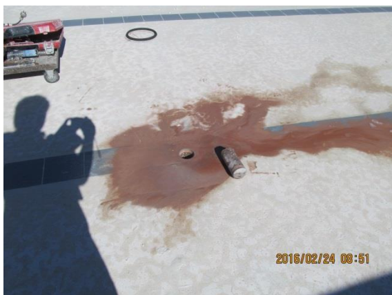
Figure B.27: The core hole at Location 6 close to the east side of the pool.
