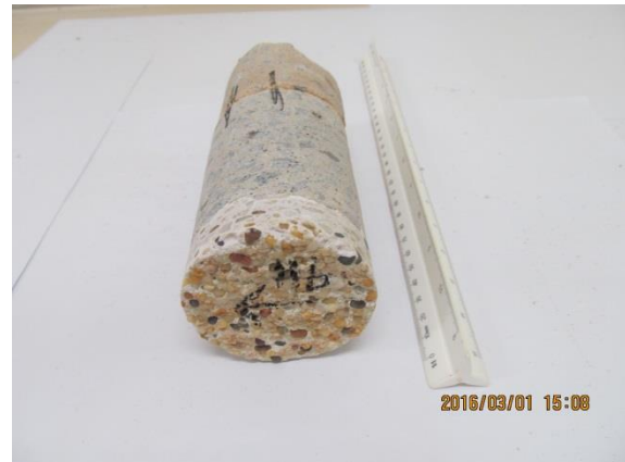
Figure 13: Core 11 Splash zone sample showing only the stone topping over the core.
