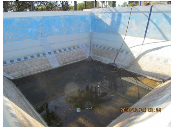
Figure B.4: View of the dive pool from north end standing inside the pool.
