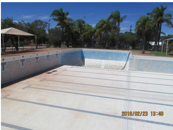
Figure B.5: View of the pool from the close to the north west corner.
