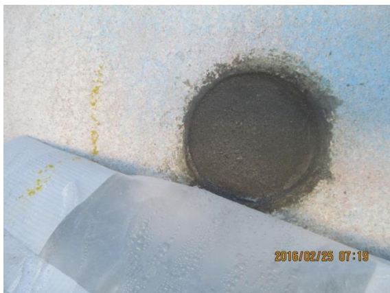
Figure B.33: Repaired core hole 7 after curing overnight.
