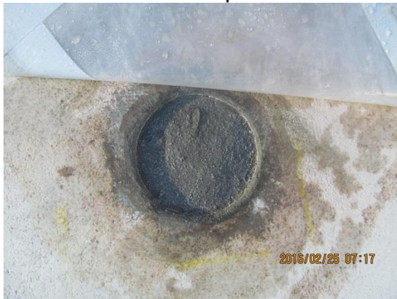
Figure B.21: Repaired core hole 4 after curing overnight.
