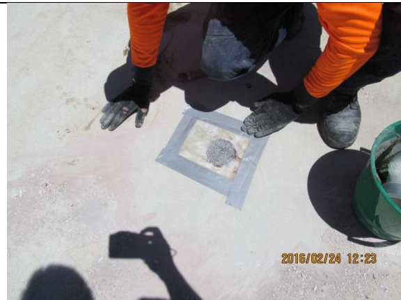
Figure B.38: Repaired core hole 8 taped over with polythene sheet.
