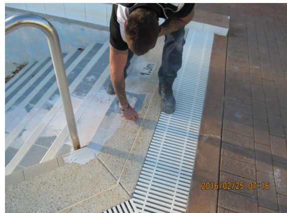
Figure B.18: Repaired core hole 3 taped over with polythene sheet.
