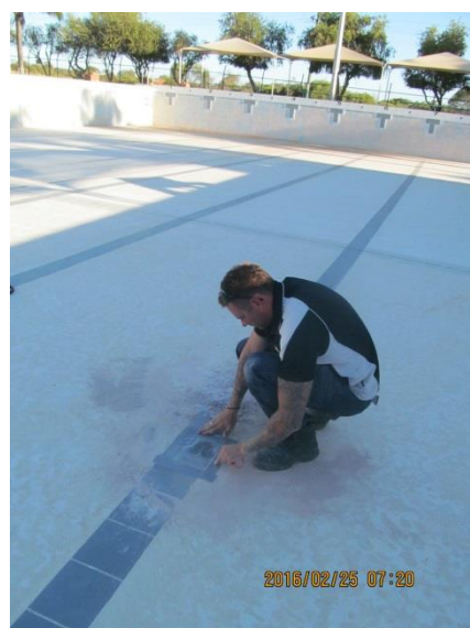
Figure B.30: Repaired core hole 6 taped over with polythene sheet.
