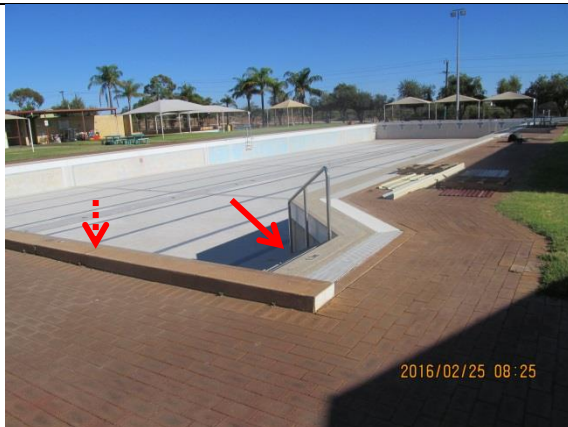
Figure 1: The south east corner of the pool (shallow end) showing the top of the stairs into the pool (solid arrow). The starter block is indicated by the dotted arrow.
