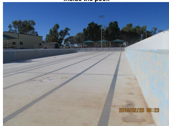
Figure B.6: View of the pool standing inside the pool at the north west corner.
