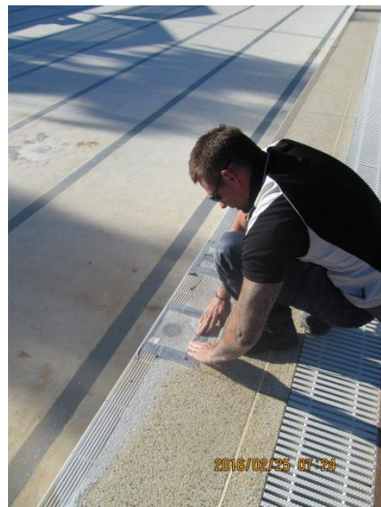
Figure B.46: Repaired core hole 10 taped over with polythene sheet.
