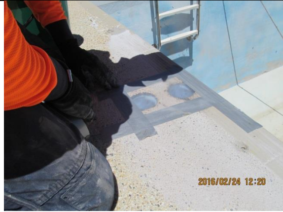
Figure B.50: Repaired core hole 11 taped over with polythene sheet.
