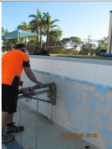
Figure B.31: The core hole at Location 7 on the east side of the pool.
