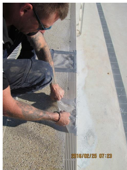
Figure B.42: Repaired core hole 9 taped over with polythene sheet.
