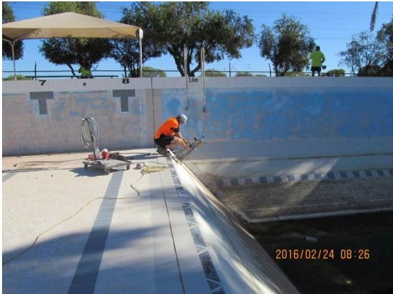
Figure B.51: The core hole at Location 12 on the sloped floor of the dive pool.
