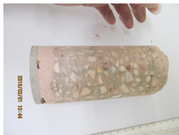
Figure 7: Core 6 Floor with a tile and intermediate material over the concrete and multi-coloured aggregates. The orange colour of the core is debris from drilling that had dried onto the core surface.
