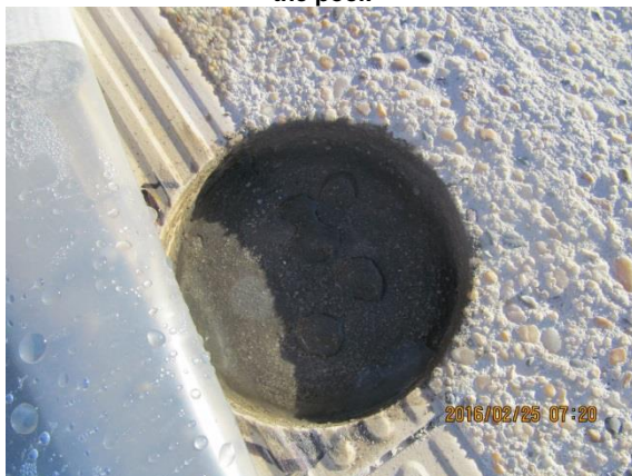
Figure B.9: Repaired core hole 1 after curing overnight.
