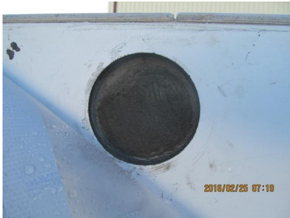
Figure B.25: Repaired core hole 5 after curing overnight.
