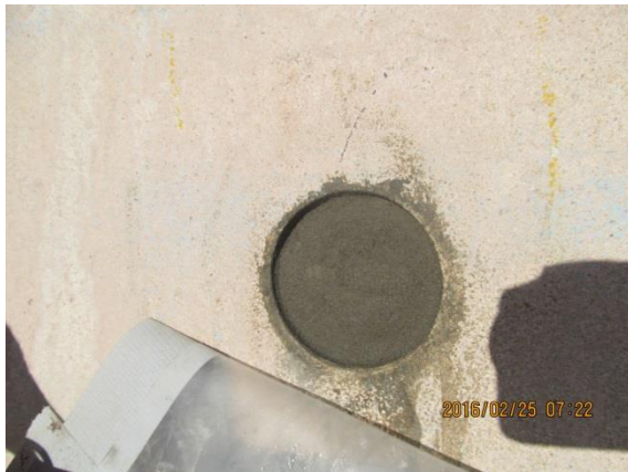
Figure B.57: Repaired core hole 13 after curing overnight.
