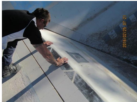
Figure B.54: Repaired core hole 12 taped over with polythene sheet.
