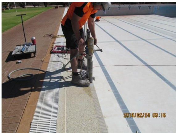
Figure B.39: The core hole at Location 9 on the west side of the pool.
