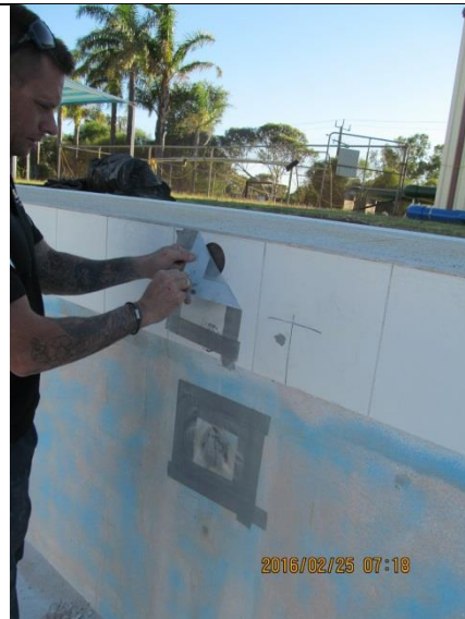
Figure B.26: Repaired core hole 5 taped over with polythene sheet.
