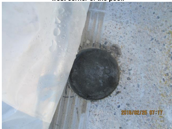
Figure B.17: Repaired core hole 3 after curing overnight.
