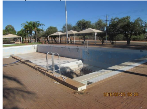
Figure B.2: View of the dive pool from the east side.
