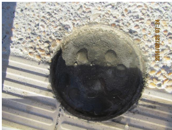
Figure B.45: Repaired core hole 10 after curing overnight.
