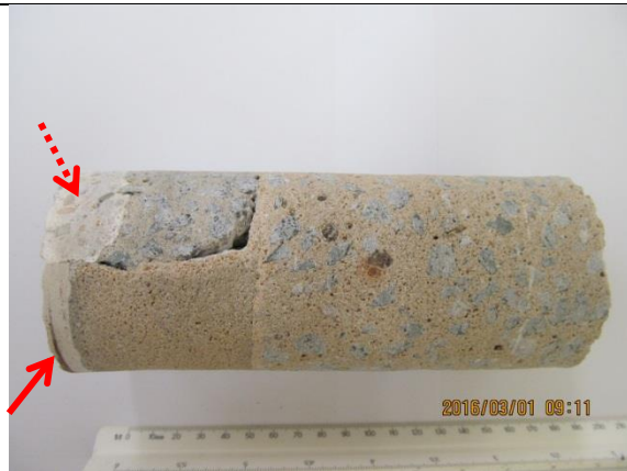
Figure 10: Core 1 Splash zone sample had both a tile (solid arrow) and a stone topping (dotted arrow) over the core. There is an intermediate material and concrete beneath the tile and stone topping respectively. A second type of concrete is observed beneath both.
