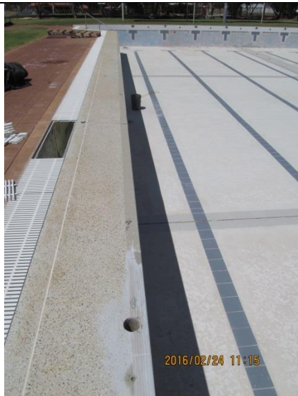
Figure B.7: The core hole at Location 1 on the east side of the pool.
