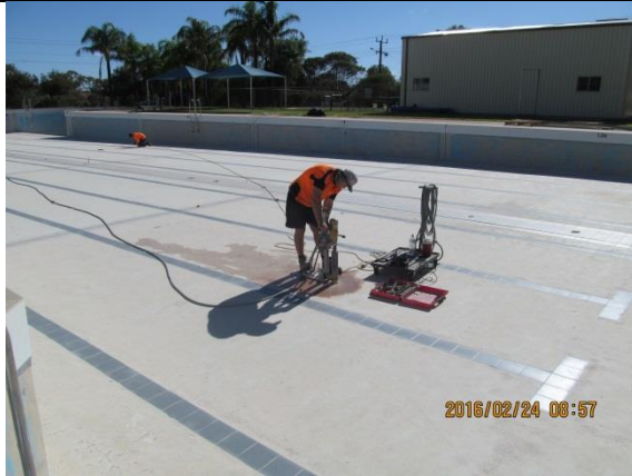
Figure B.19: The core hole at Location 4 on the south west of the pool.
