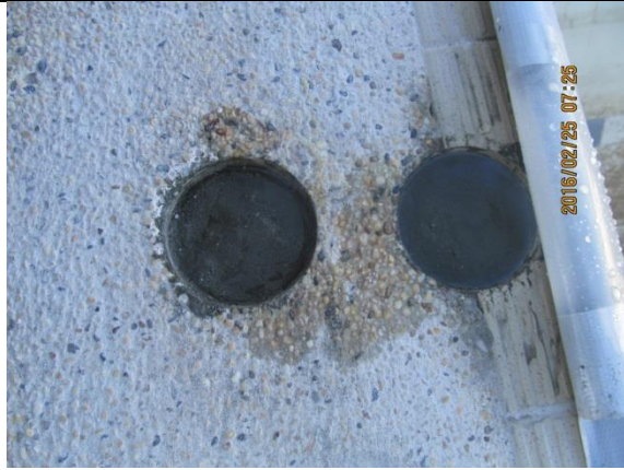
Figure B.49: Repaired core hole 11 after curing overnight.
