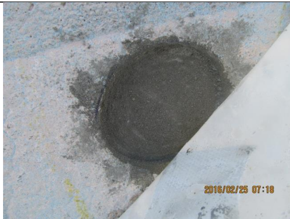
Figure B.13: Repaired core hole 2 after curing overnight.
