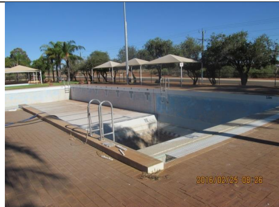
Figure 2: The dive pool area on the north east side of the pool.
