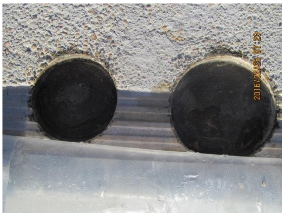
Figure B.41: Repaired core hole 9 after curing overnight.
