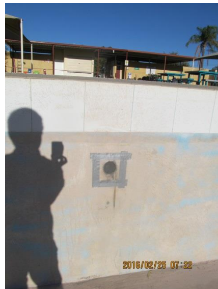
Figure B.58: Repaired core hole 13 taped over with polythene sheet.
