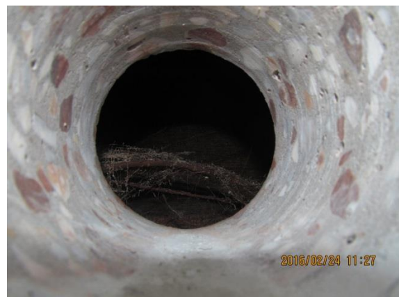
Figure 4: Core hole 13 (Beneath the splash zone) with a void at approximately 150 mm from the surface of the pool wall.
