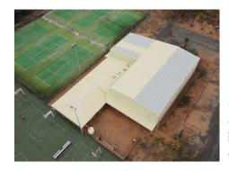
Plans to replace the recreation centre roof have been accelerated with the availability of Federal Government funding. The roof is nearing 40 years of age and water ingress is threatening to cause internal corrosion and damage to the basketball court floor.
