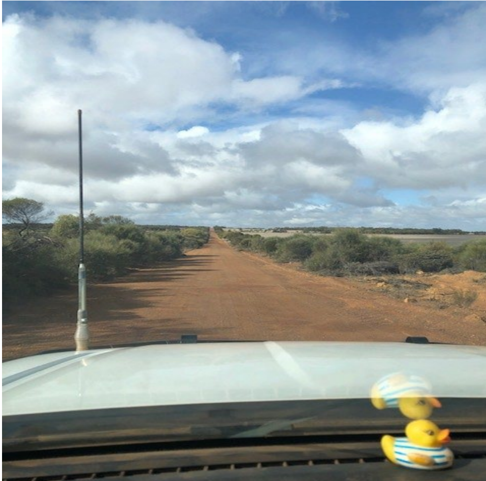
Figure 4 Streets at slk 0.31 vegetation extending over road reducing safe travel surface to 4.0 m.
