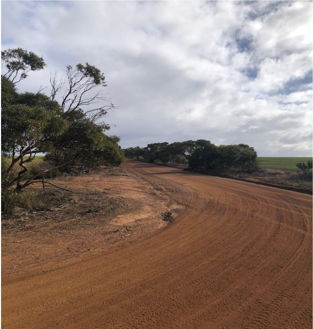
Figure 6 Streets Road at 2.4 m height of truck as per assessment requirements. Tyre marks indicate full road taken up when heavy vehicle turning.
