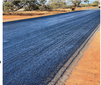
Right: Morawa-Yalgoo Project Works
