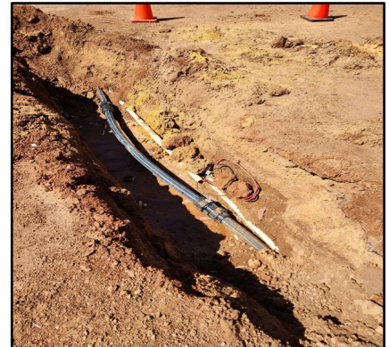
Right: Townsite Drainage Works
