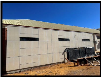
Left: Works progress on Town Hall Storage Area.
