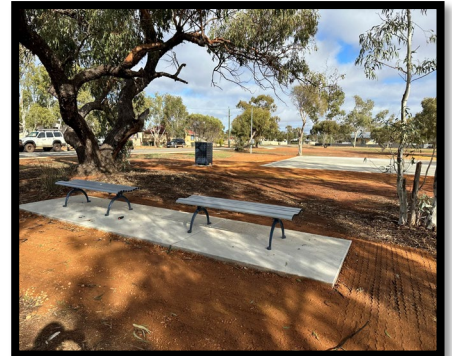
Right: Work Progress on Wildflower Park
