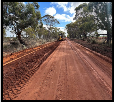
Left: Works progress on Milloy Road
