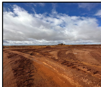
Right: Work progress on Landfill
