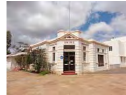
PHOTO 27 - MORAWA SHIRE OFFICE
