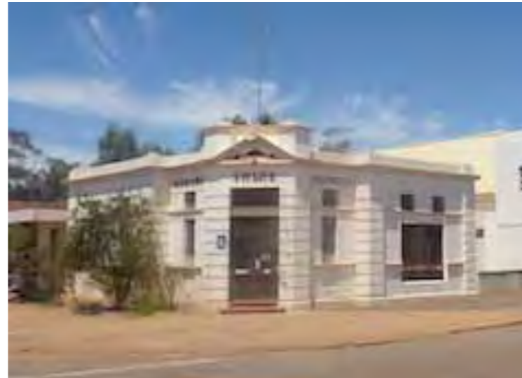
PHOTO 1 - MORAWA SHIRE OFFICE
