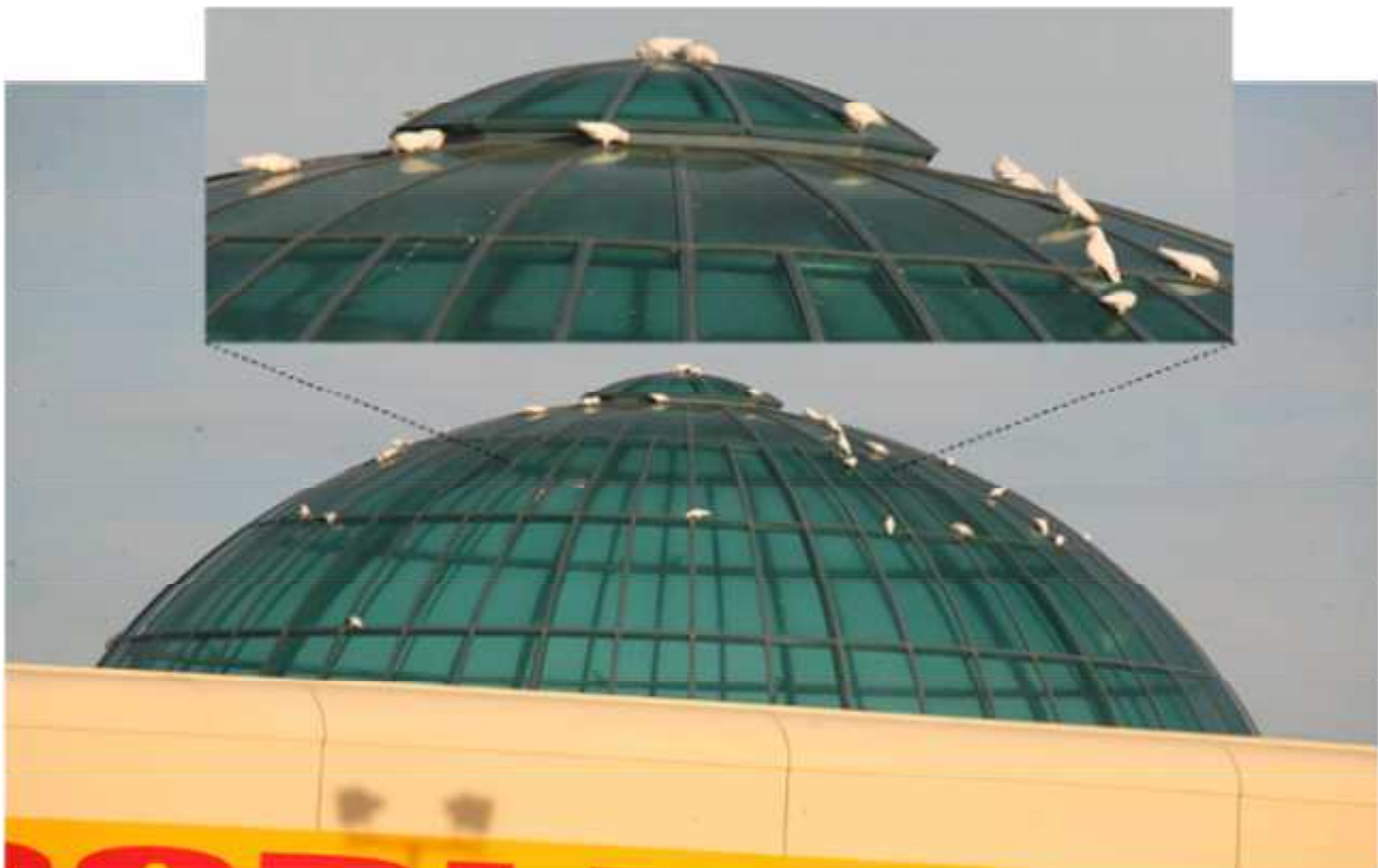
Figure 2. Glass dome on shopping centre at Seaford, with Little Corellas picking at rubber seals between the glass panels, February 2010.
