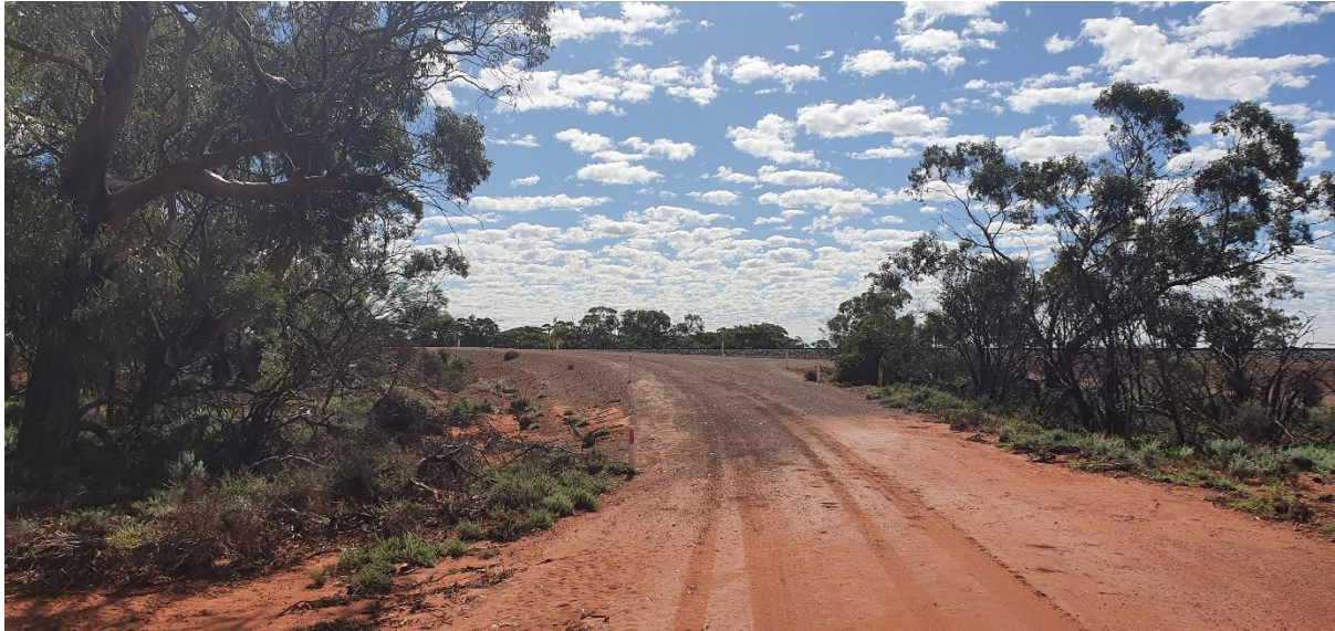
Finding 2.7 – Poorly delineated curve on approach to rail crossing on Ross Road
