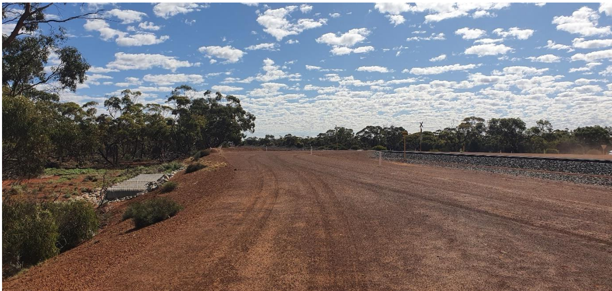
Finding 2.4 - Culvert and steep embankment in clearzone on Ross Road
