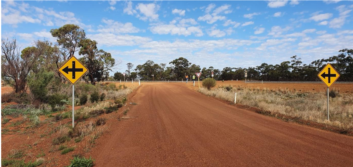
Finding 2.3 – Non-Standard Advanced Intersection Warning Signs
