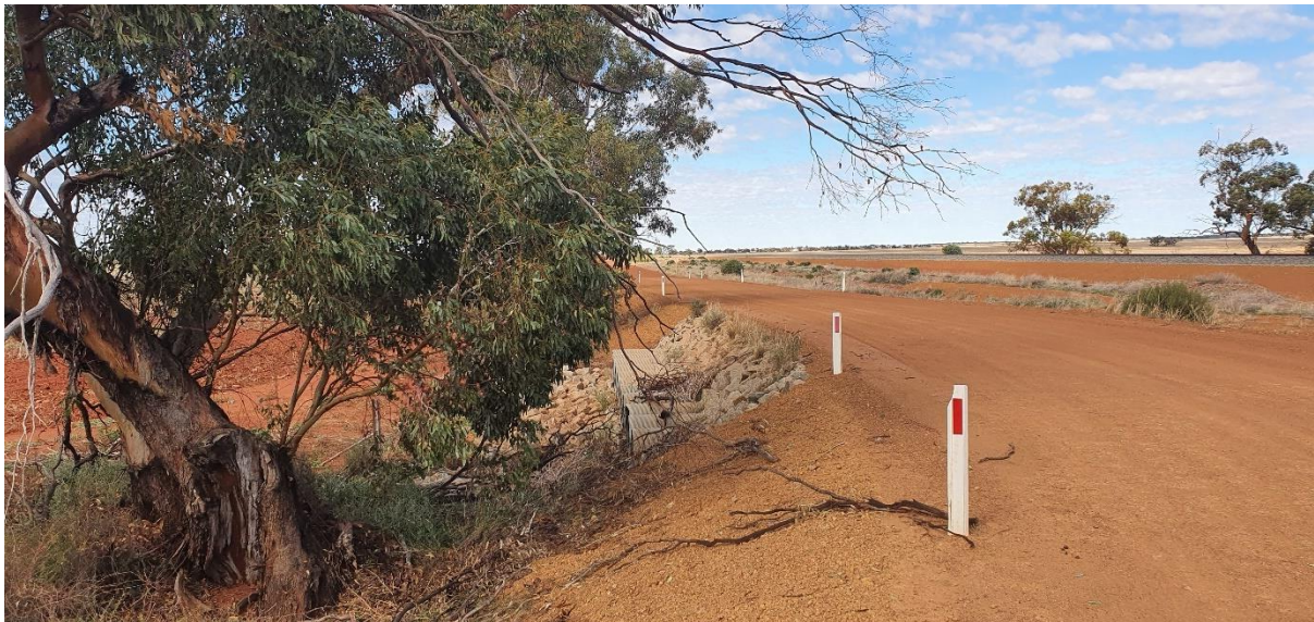
Finding 2.4 Culvert and rock pitching in clearzone
