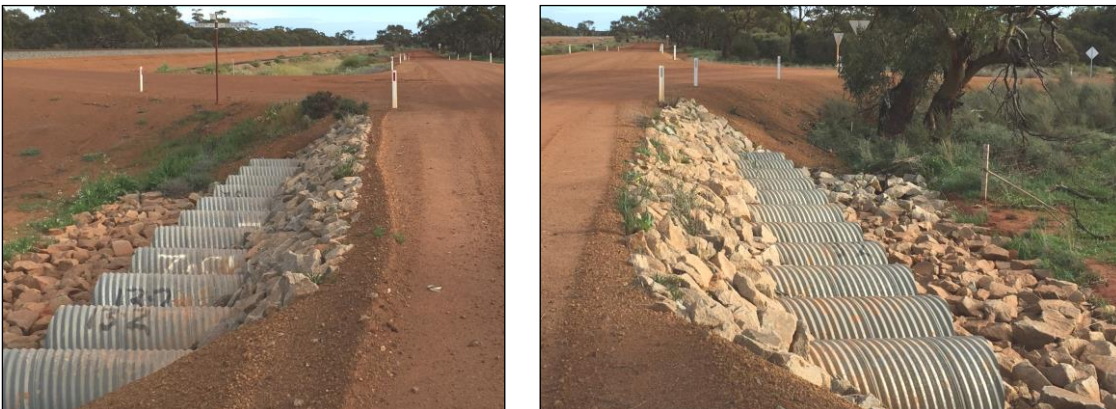
Figure 1 Rock protection around Culvert 2 (11xØ900mm CSP) inlet and outlet
