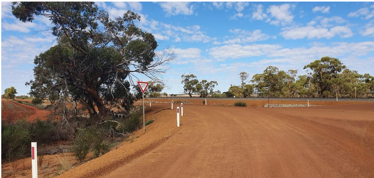
Finding 2.2 – Steep Embankment at side of Stephens and Evaside Road
