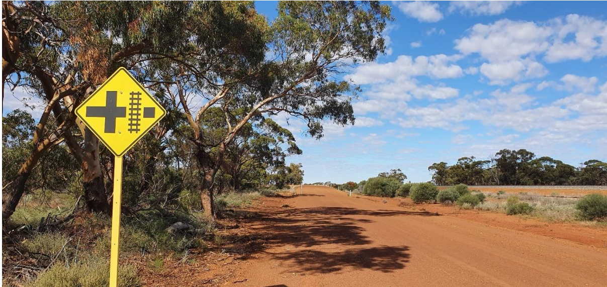
Finding 2.8 – Restricted sight distance over crest prior to intersection north bound on Evaside Road
