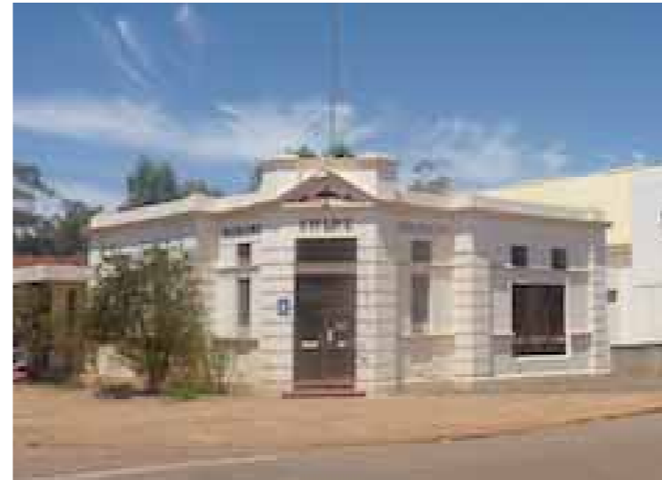
PHOTO 1 - MORAWA SHIRE OFFICE
