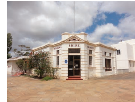
PHOTO 27 - MORAWA SHIRE OFFICE
