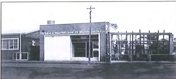
View of the Rural and Industries Bank of WA (fmr) from 1961 Source: State Library of Western Australia Ref: 006257D
