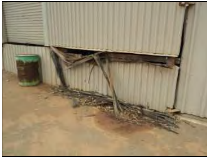
Termite damage
