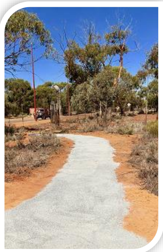
New bush trail under construction
