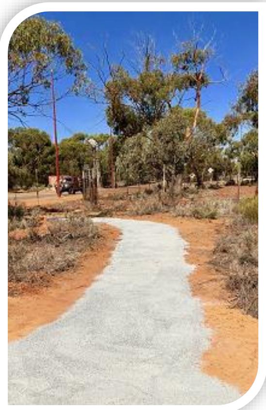
New bush trail under construction
