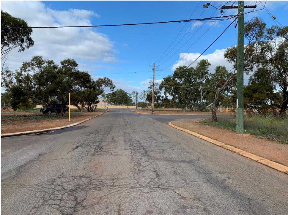
*Figure 3: Broad Av looking east from approx. S1k 0.12 showing distressed surfacing.*
