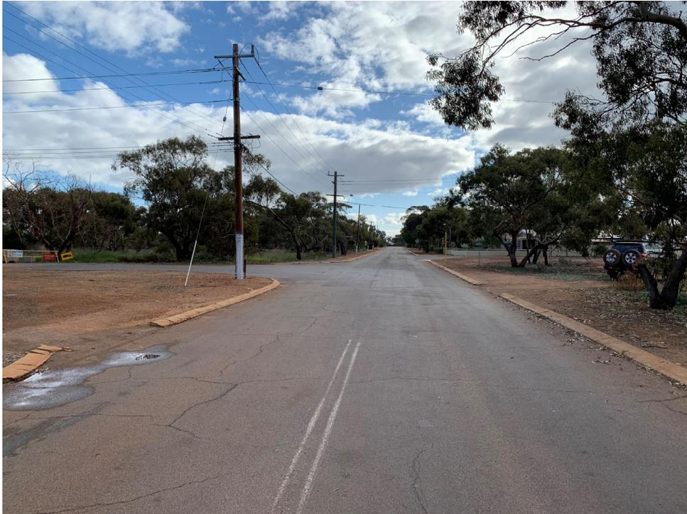
*Figure 1: Broad Av looking west from approx. Slk 0.05 showing power pole prior to the CBH intersection (LHS) and damaged kerbing.*
