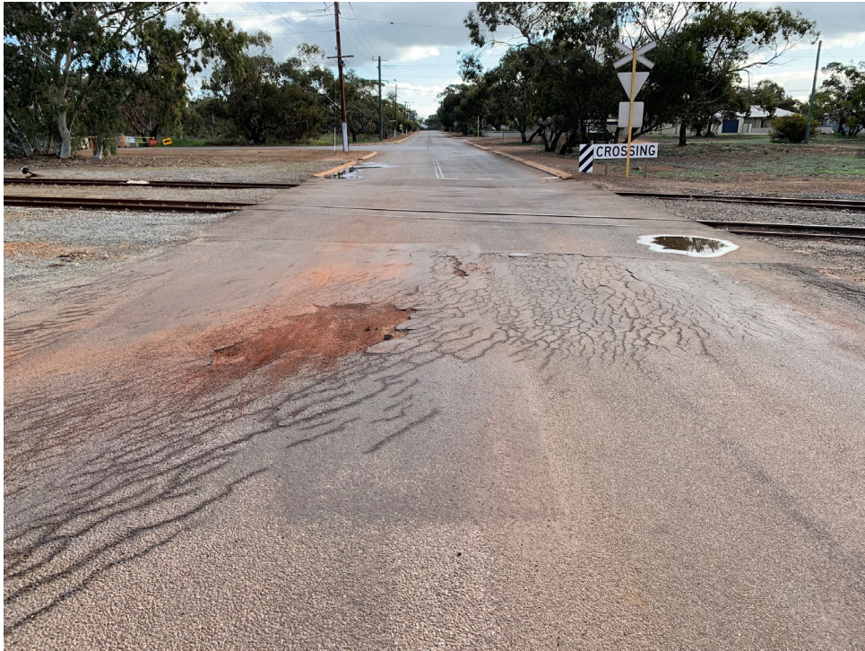
Figure 5: Broad Av looking west from approx. Slk 0.01 showing distressed surfacing and potholes east of rail spur line crossing at the Broad Av / CBH sampling station intersection.
