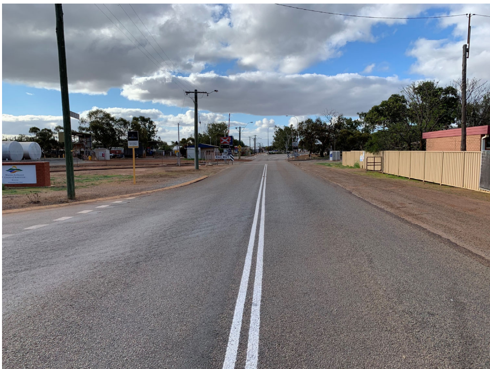
Figure 6: Wubin Mullewa Rd looking north from Broad Av intersection showing informal trafficable verge on eastern side (RHS) and power pole on western side of intersection.
